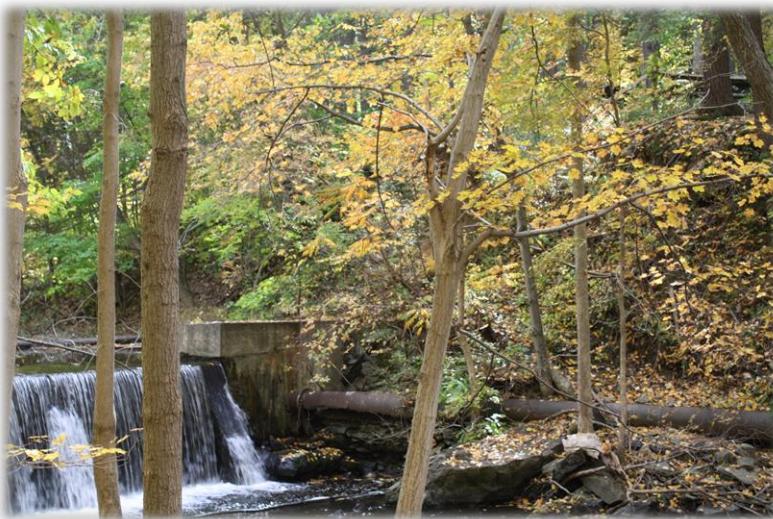
Dam on the lower Saw Kill, showing remnants of the penstock that provided water to the hydroelectric turbine near the mouth of the creek.
